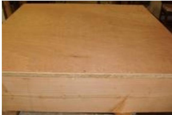
1/4" plywood underlay on sub-floor
