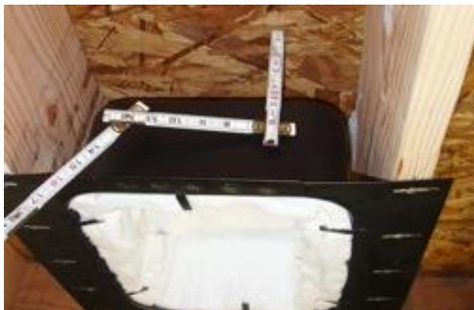
Back Box Installed showing overhead clearance
